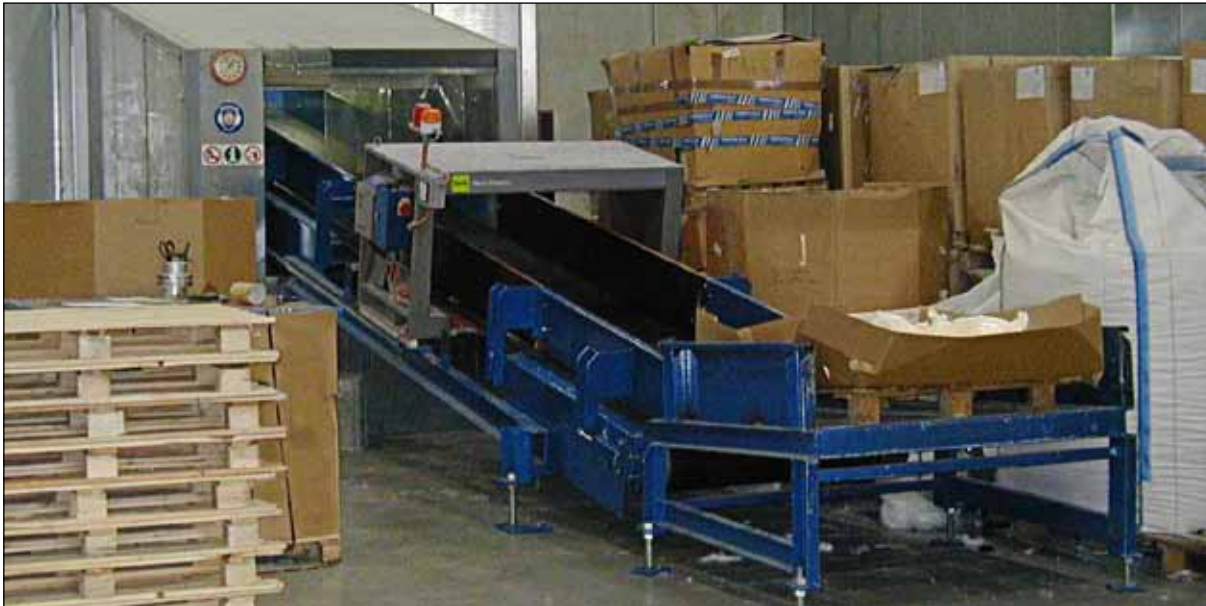
DLS tunnel metal detector inspecting for metal residues of recycling material before the mill
